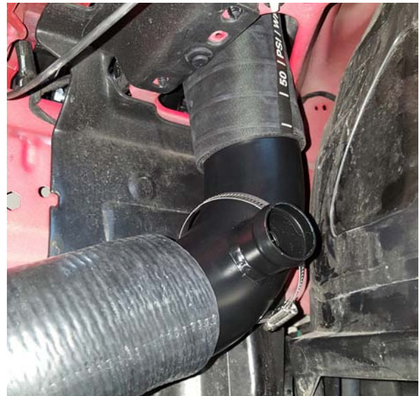
Surge Tube Installed
