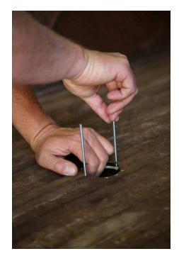
18. The studs are used as an installation tool and will be removed later during assembly.
